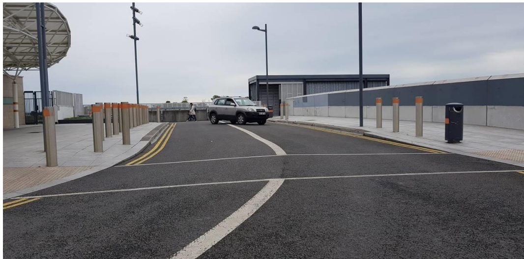
Figure 32: No Turning Circle adjacent to Railway Station entrance
