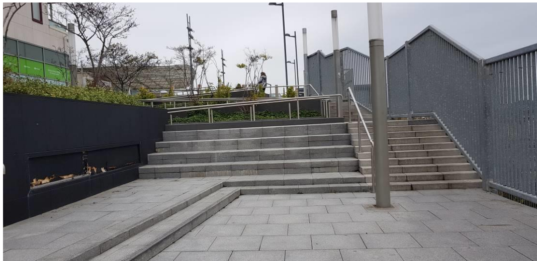
Figure 30: Lack of Tactile Guidance at steps/hazards
