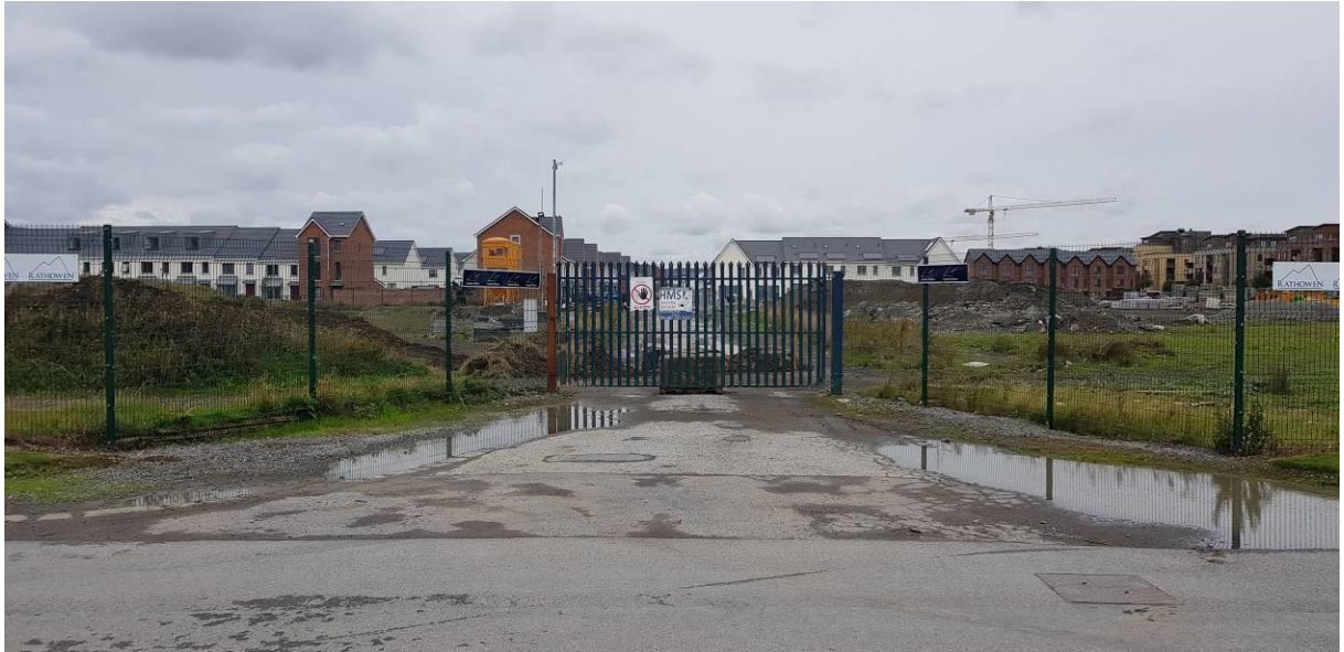
Figure 6: Ponding at Junction
