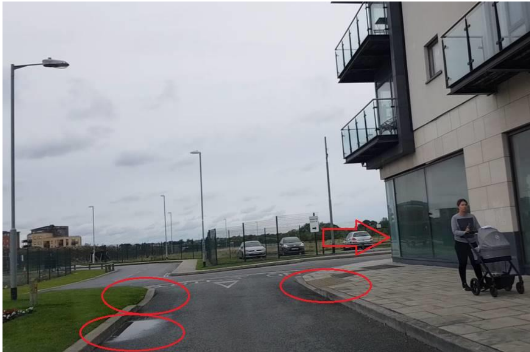
Figure 17: Building Line restricting forward visibility adjacent to Block 12 (note also ponding issues and tactile layout)
