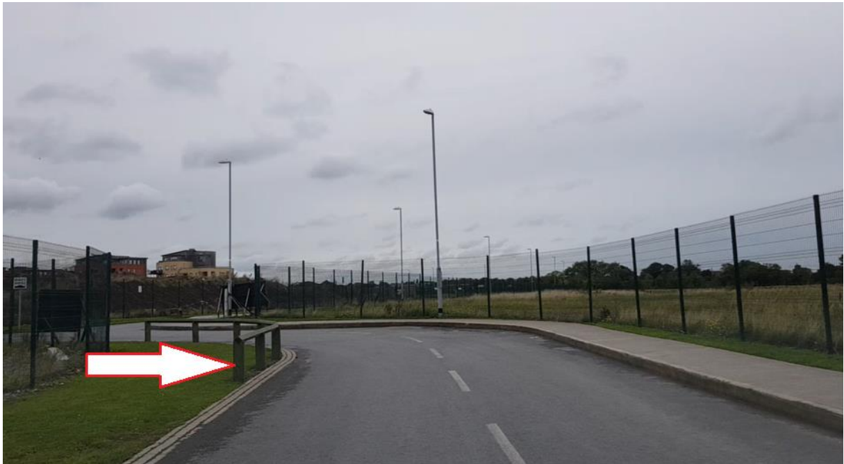
Figure 15: Fencing Located too close to carriageway (note narrow cross section on bend)
