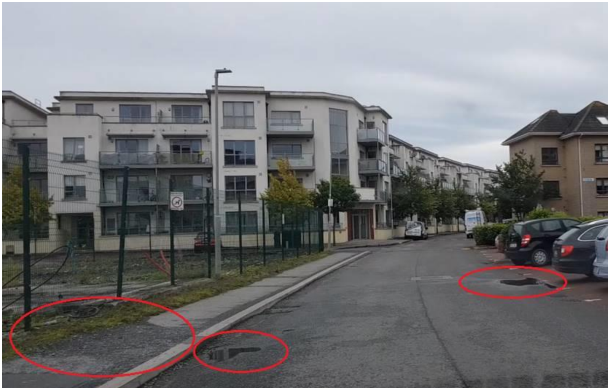
Figure 9: Debris on footways/ poor carriageway condition & ponding on Railway Rd
